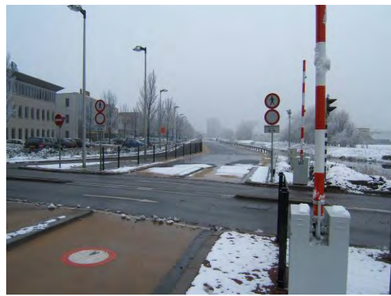
Figure 7. 2getthere's two-lane guideway with no physical barrier between lanes.
